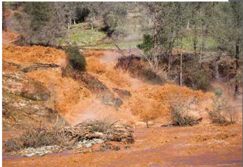
Oroville Dam Spillway Erosion, Feb. 11, 2017. Water and debris from the emergency spillway failure flow into the diversion pool just downstream of the dam. Source: Dale Kolke, DWR.
