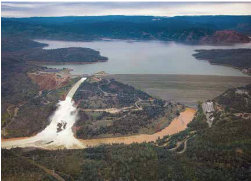
Oroville Dam's Main Spillway at 100,000 cfs. An aerial view looking eastward toward Oroville Dam and Reservoir. The emergency spillway is on the left (note eroded red dirt area) and the damaged main spillway left of center. Oroville Dam is on the right. An outflow of 100,000 cfs travelled down the main spillway on Feb. 15, 2017. Source: Dale Kolke, DWR.
