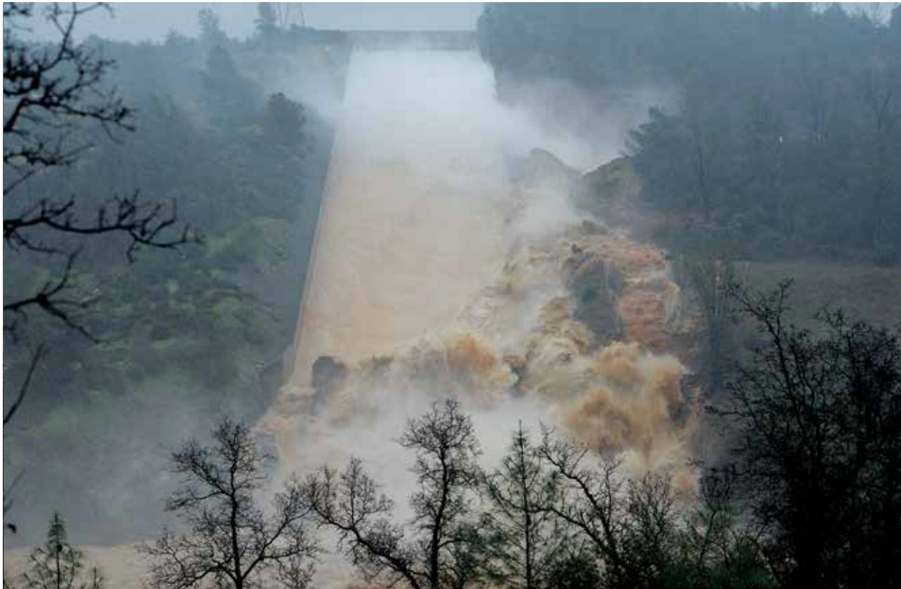
The Oroville Incident, Feb. 2017. As the Oroville Reservoir main spillway crumbles, mud, rocks and concrete flow in to the Feather River on February 8, 2017. Source: Bill Husa, Chico Enterprise-Record .
