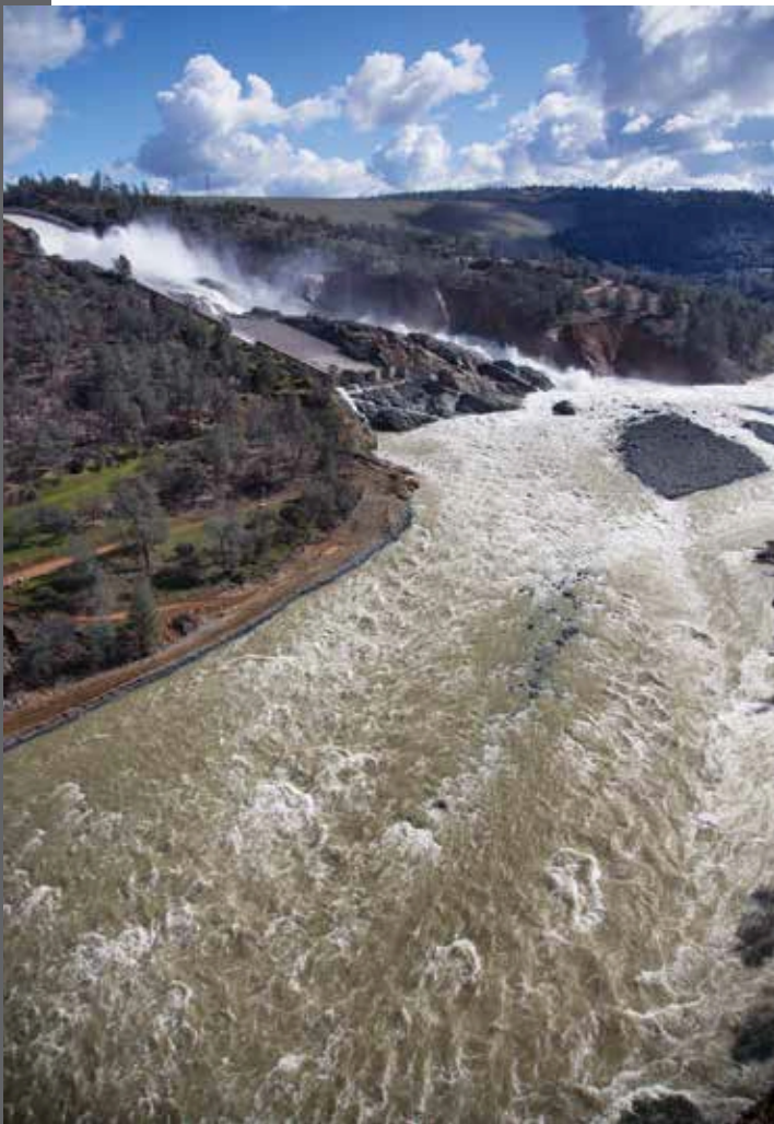
An aerial view of the diversion pool on the Feather River as outflow from the damaged Oroville Dam spillway was being reduced from 50,000 cubic feet per second (cfs) to zero on February 27, 2017. Source: Dale Kolke / California Department of Water Resources
